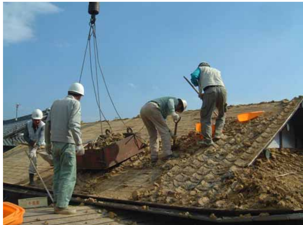
Before (改修前) - 屋根改修 -
